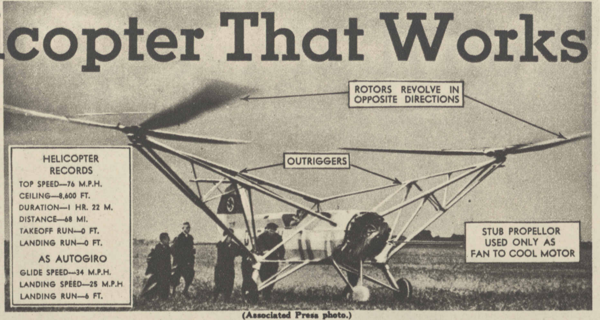
The Focke helicopter at rest after one of its experimental flights. No attempt has been made as yet to cover the outriggers or to streamline the plane in order to increase the efficiency of its performance.
