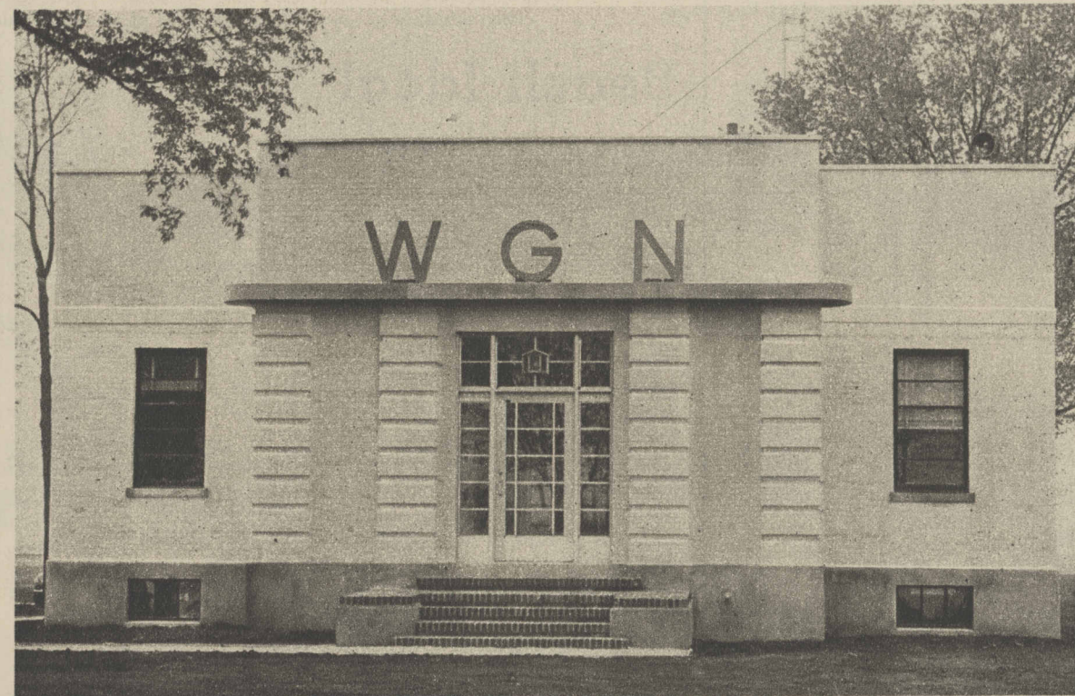
Front view of the transmitter house, in which are located instruments pictured on this page.
