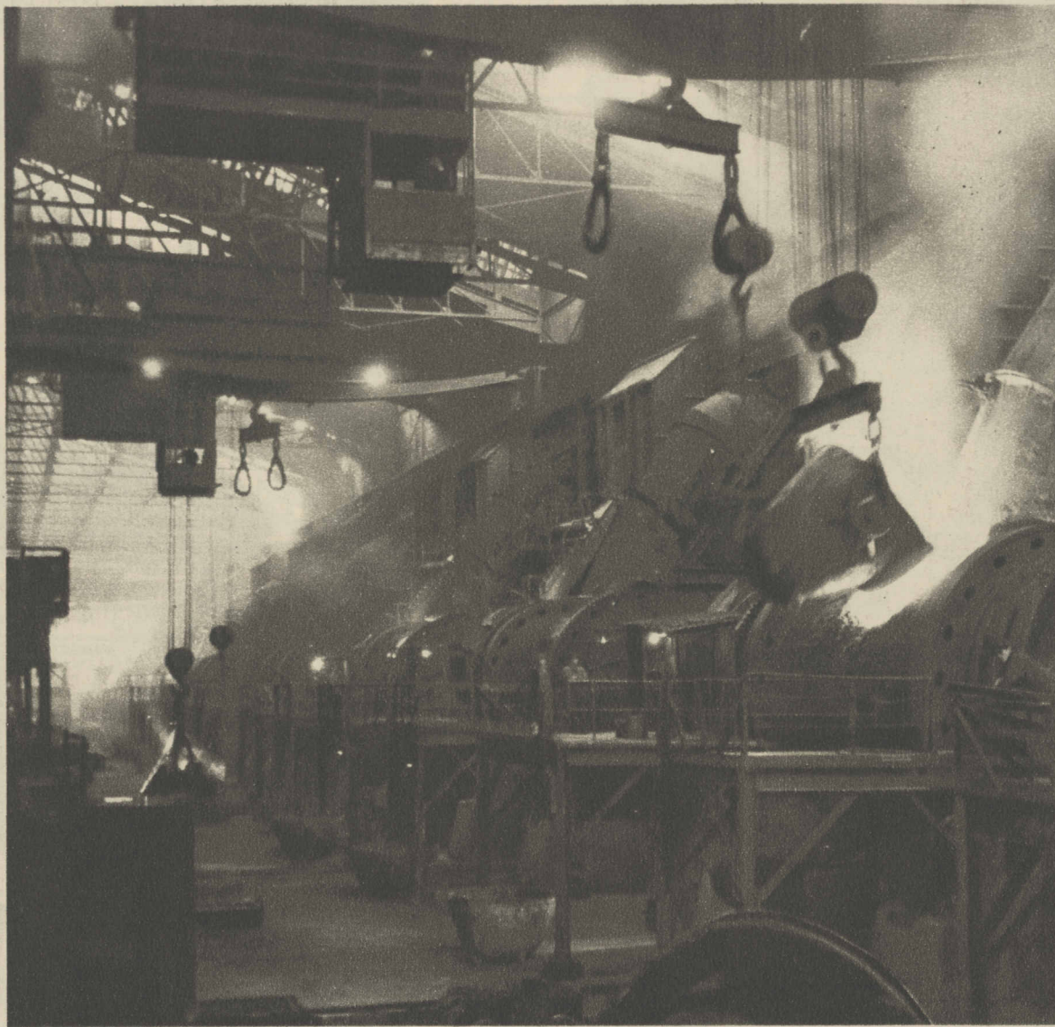
Aile of converters in Canadian smelter where more than 90 per cent of world's supply of nickel is produced. (Thomas photos, courtesy International Nickel Co., Inc.)
