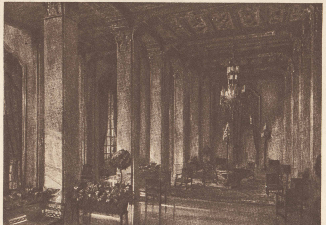
VIEW OF NORTH LOBBY—HOTEL SHORELAND
