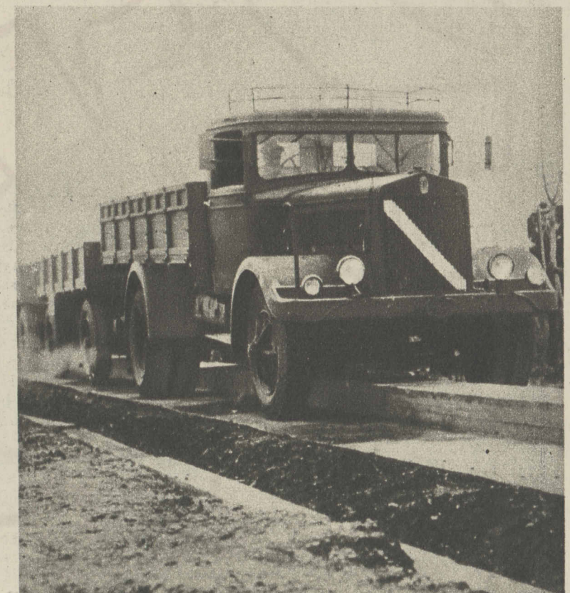
Italy tries out a new military idea—an experimental highway featuring a "third rail," or center ramp that guides a power lorry and its long train of supply-carrying trailers.
