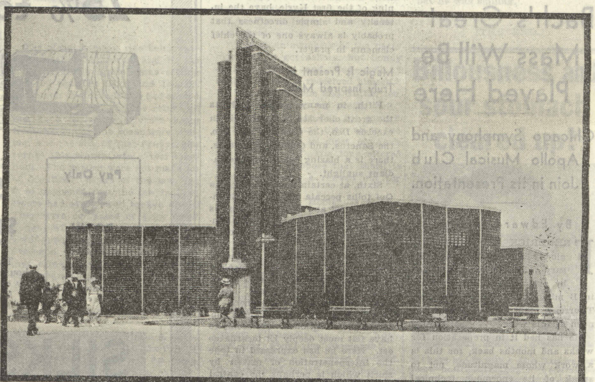
Perhaps the newest of all building materials is glass brick. The building pictured here, an exhibit at the Chicago World's Fair, was made entirely of glass.
