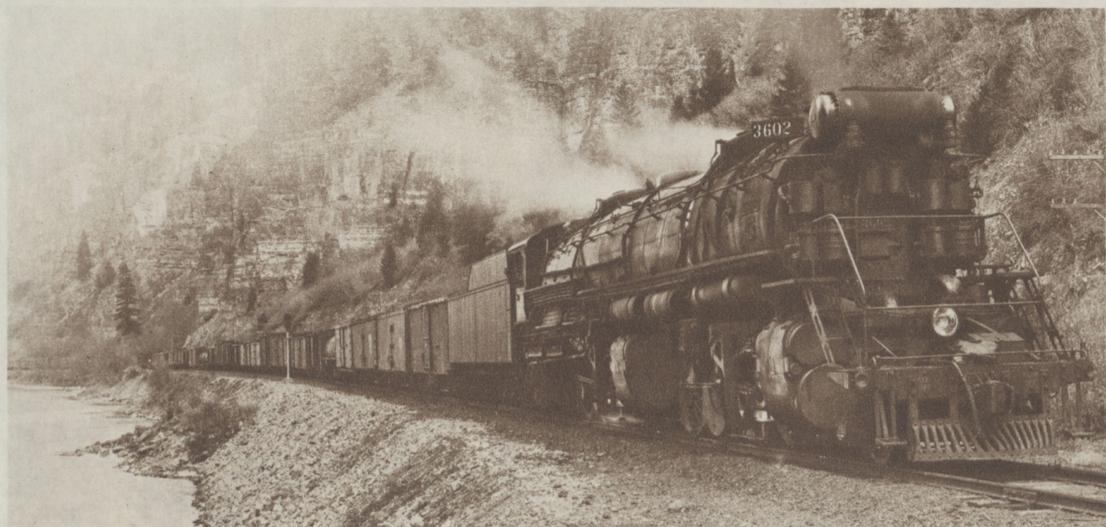
A NEWLY DEVELOPED AIR BRAKE makes 150-car freight trains, operating at passenger-train speed, as easily handled as a small auto. This train, whose cars are among the 1,000 already equipped with the new brakes, is hauled by a locomotive with sixteen driving wheels.
