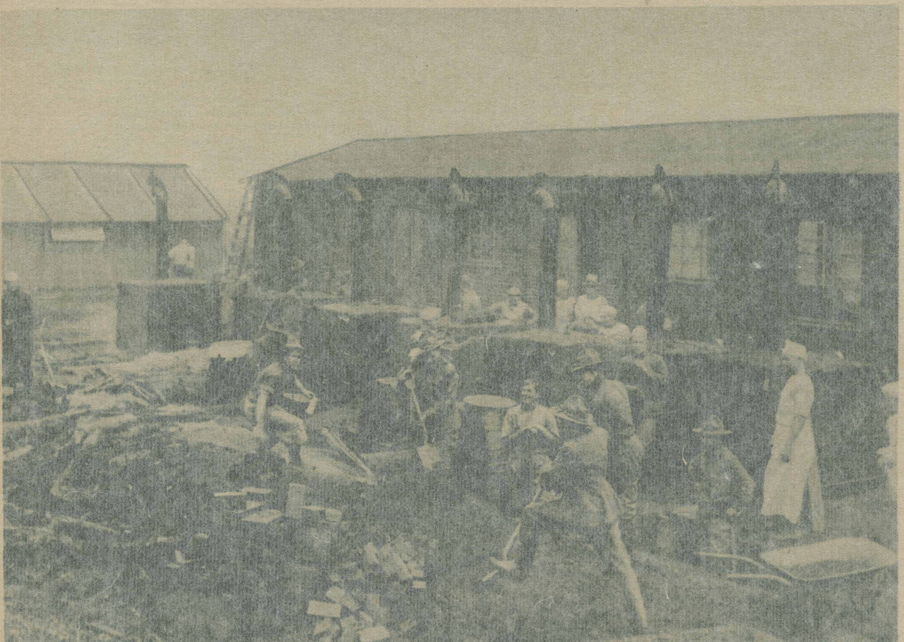
BUILDING MORE BAKE OVENS AT THE AMERICAN CAMP IN FRANCE—The boys appear, from this picture, to be in good spirits and indications are that they are well housed and fed.
