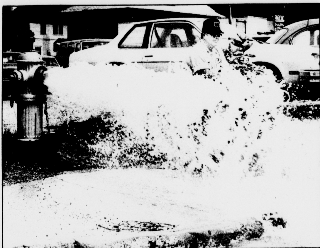
Bud Curtis, with the City of East Lansing Water Department, is flushing the hydrant at Division Street between Albert and Grand River avenues of lime. It takes about two hours and is done once a year.
