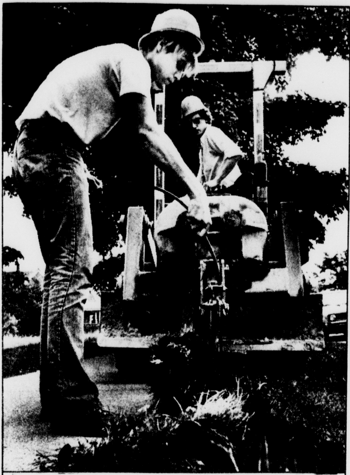
State News/Deborah J. Borin Dave Biergans is plowing the cable line, while Roger Olmstead lays the new cable along Grand River Avenue. Newly installed trees damaged the cables to street lights at Collingwood Drive and Grand River Avenue.
