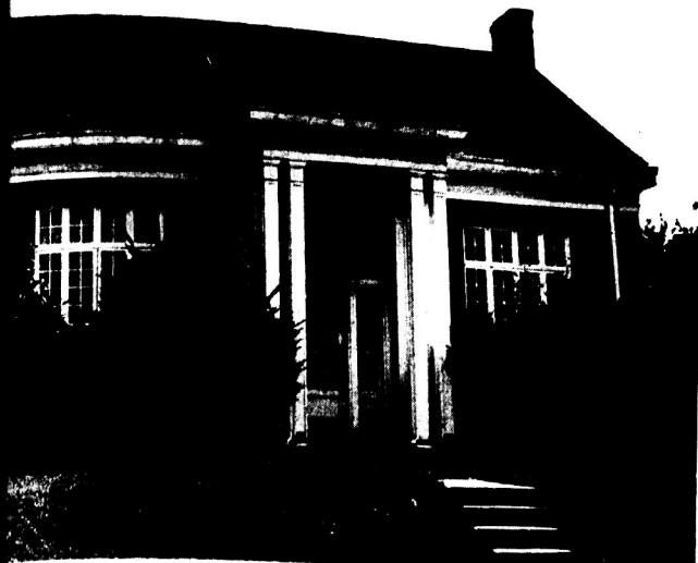
Orchard Street Pumphouse
