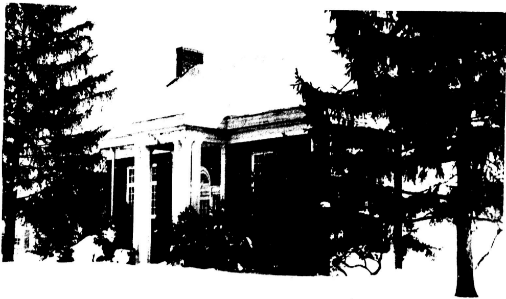
The pump house on Orchard Street in East Lansing.
