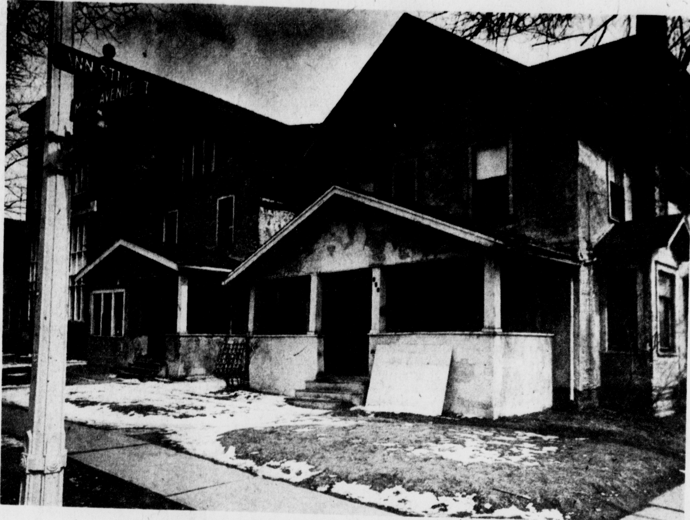
These two houses at the corner of M.A.C. Avenue and Ann Street will be torn down to make way for a 24-hour restaurant, offices and student apartments. The developer says that the complex will benefit the community, despite protests from area residents. SN photo/Bob Kaye
