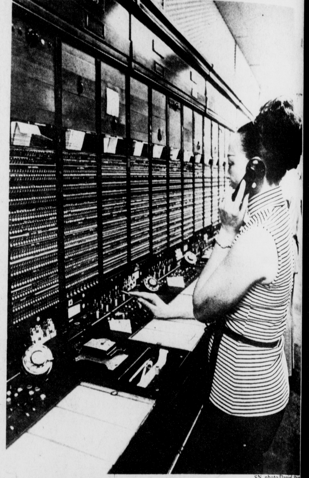
Cleo McFadden, asst. manager of Operator Service, takes a long distance telephone call from a coin operated booth, performing an important function which can not be done by machines. To the left is a calculagraph a device that is used for timing such calls.
