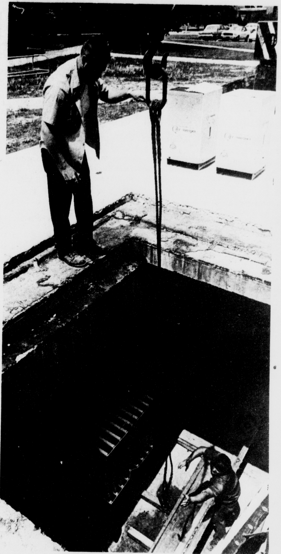
Larry Swain, top, and Ronald Antcliff below, from Superior Electric, Lansing, install a new 13,000 volt service into the Physics and Astronomy Building near lot G Monday.
