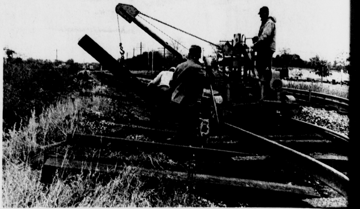
Working on the railroad
