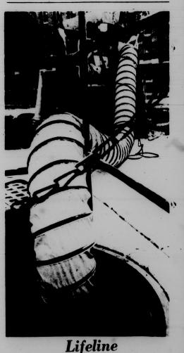
This snake-like device provides cool air and oxygen to the workmen below, who are hooking up telephone lines for the new library addition.
