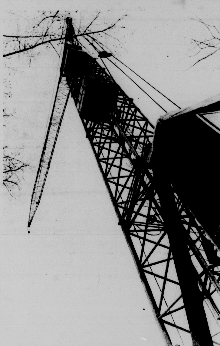
HIGH LIFT crane being used on the Kedzie construction job cost $100,000 and rents for $35 per hour. It has a 98-ft. boom and takes four days to set up. Photo by Cal Crane
