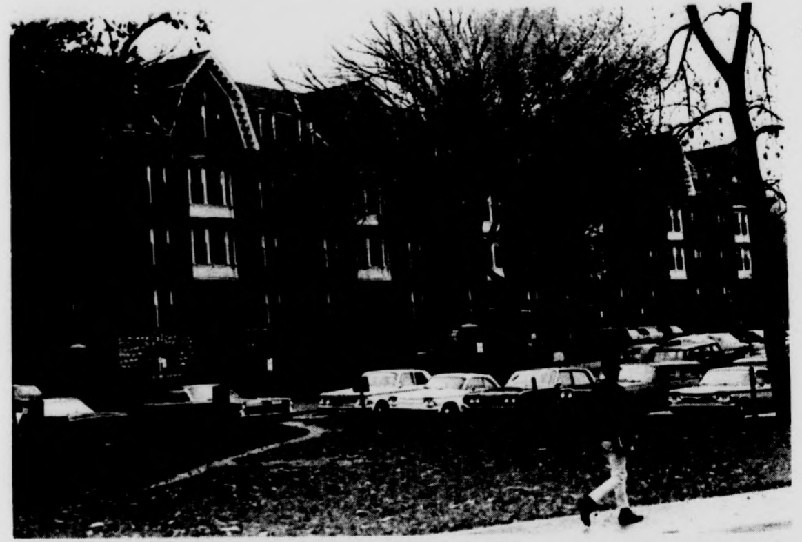
BEFORE--Wells Hall was one of the oldest buildings on campus, built in 1905 as a men's residence hall. It later served as an office building for faculty members from various colleges. In 1966 it was torn down to make way for a graduate-library addition to the Library. Photo by Russ Steffey
