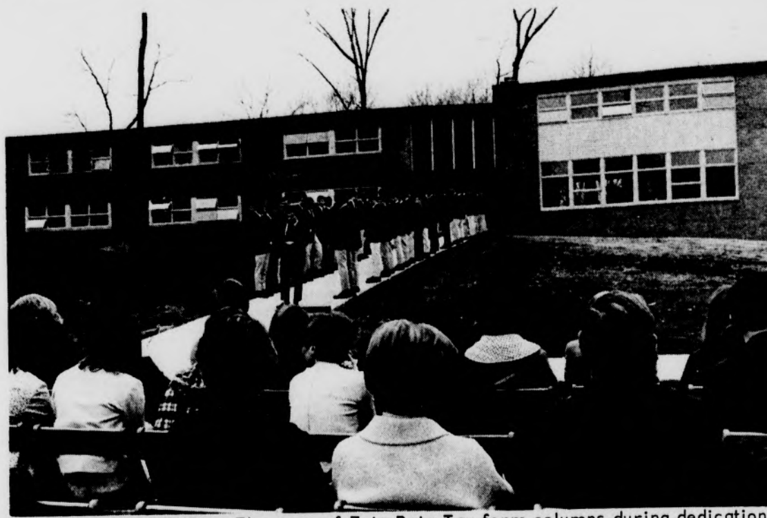
THEY DID RETURN--The men of Zeta Beta Tau form columns during dedication ceremonies of their renovated house. They had been living around East Lansing since the house was burned in February of 1965. Photo by Jonathan Zwickel
