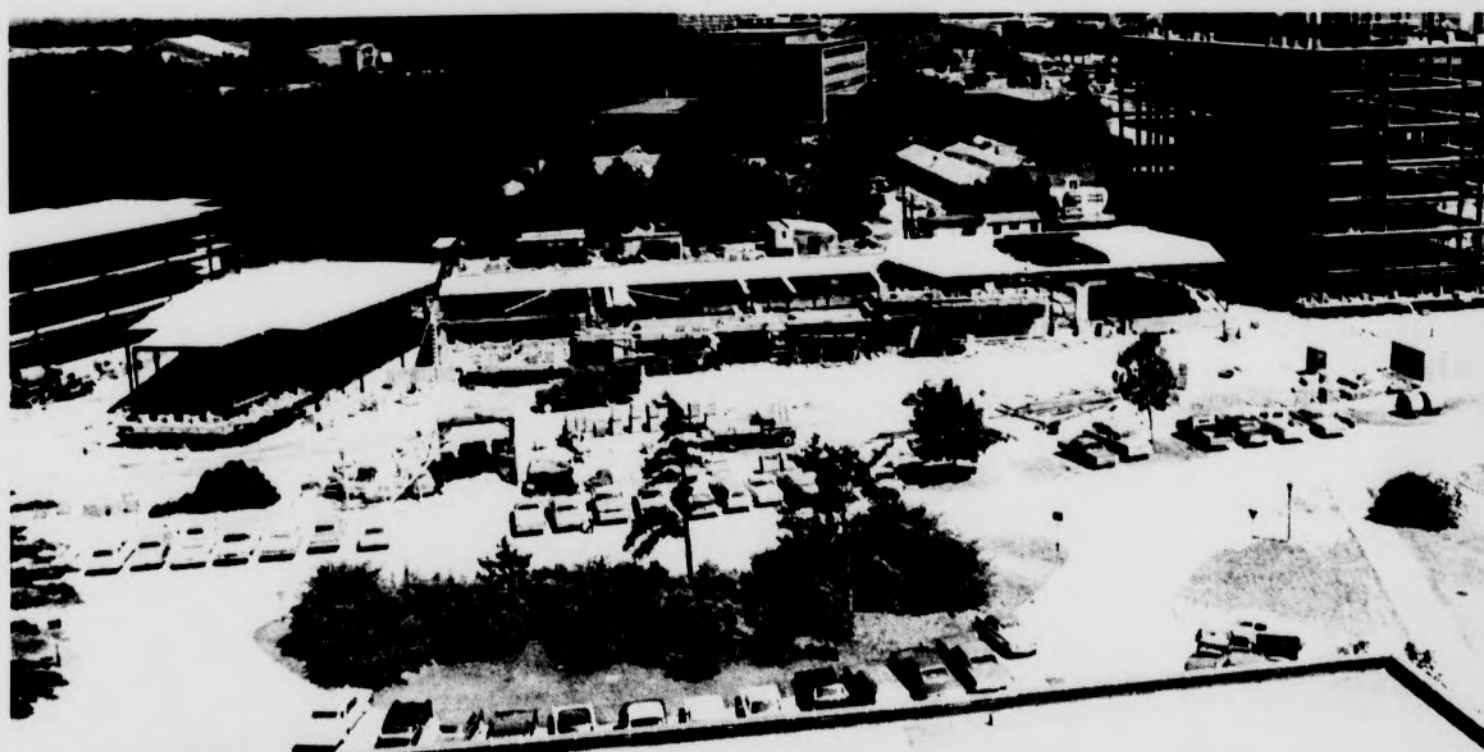
FOREIGN FLAVOR AND EQUATIONS--Next door to the International Center is an appropriate spot for this campus addition--the Language and Mathematics Building. It is scheduled for completion in March 1967.
