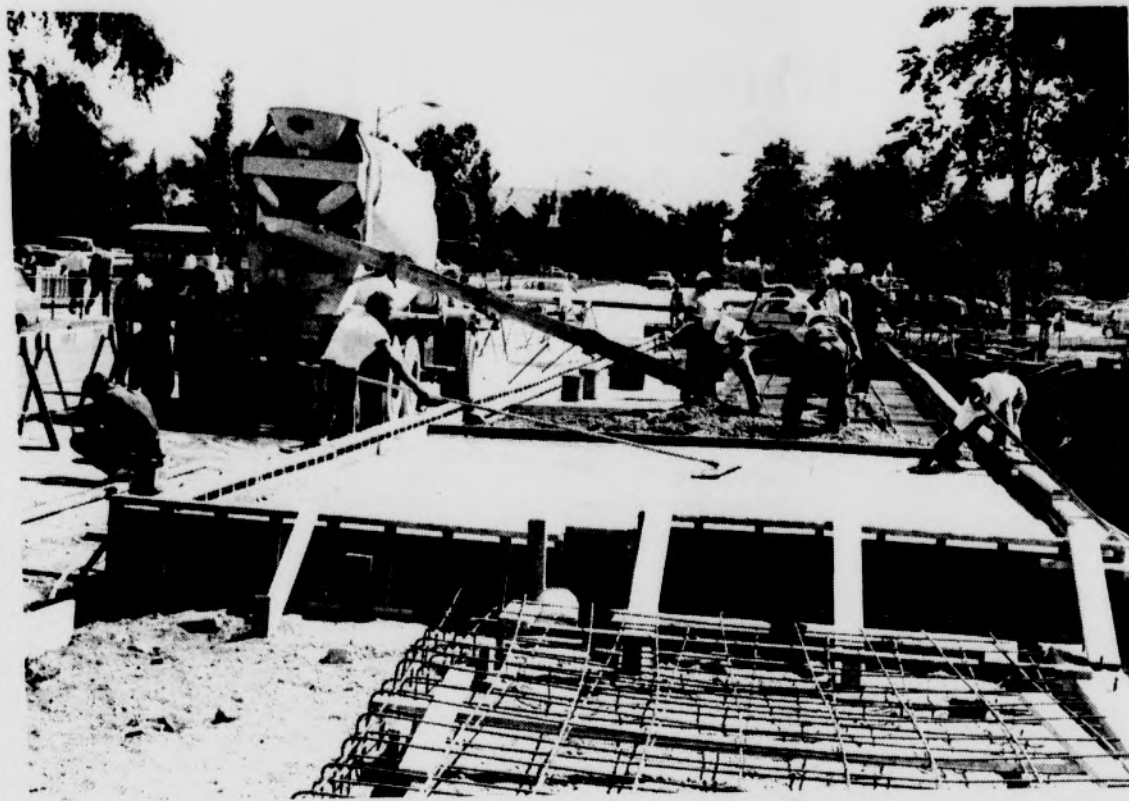
Bridge Over The River. . .
