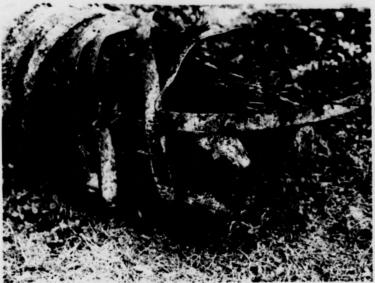
CAMPUS PIPELINE -- Pipe construction has changed a lot since the old wooden pipe with iron bands was placed under West Circle. It is being replaced by the three pipes at right.
