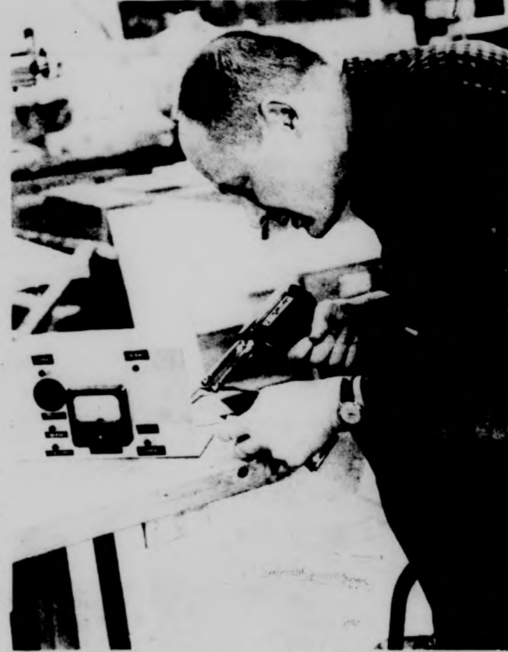
PSYCHOLOGY ISN'T ALL TESTS AND THEORY-- Royal Olson repairs a soldered joint on an instrument that measures the reactions of a Pavlov dog. The dog is trained to drool in reaction to a bell and lights as it would to meat. Photo by Russell Steffey
