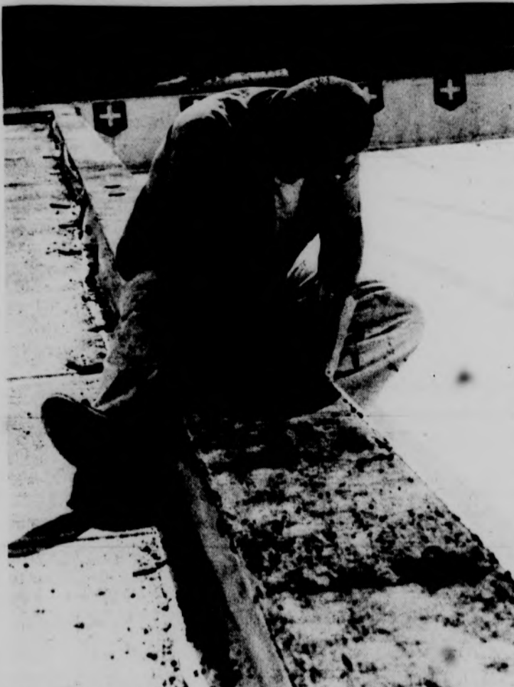
THE HEAT IS ON--Warm weather has come to campus, and with it has come the longing for spending sunny afternoons at the IM pool. Unfortunately, workmen such as this one are still preparing the pool for use. No date at which the pool may be used has yet been announced. Photo by Jonathan Zwickel
