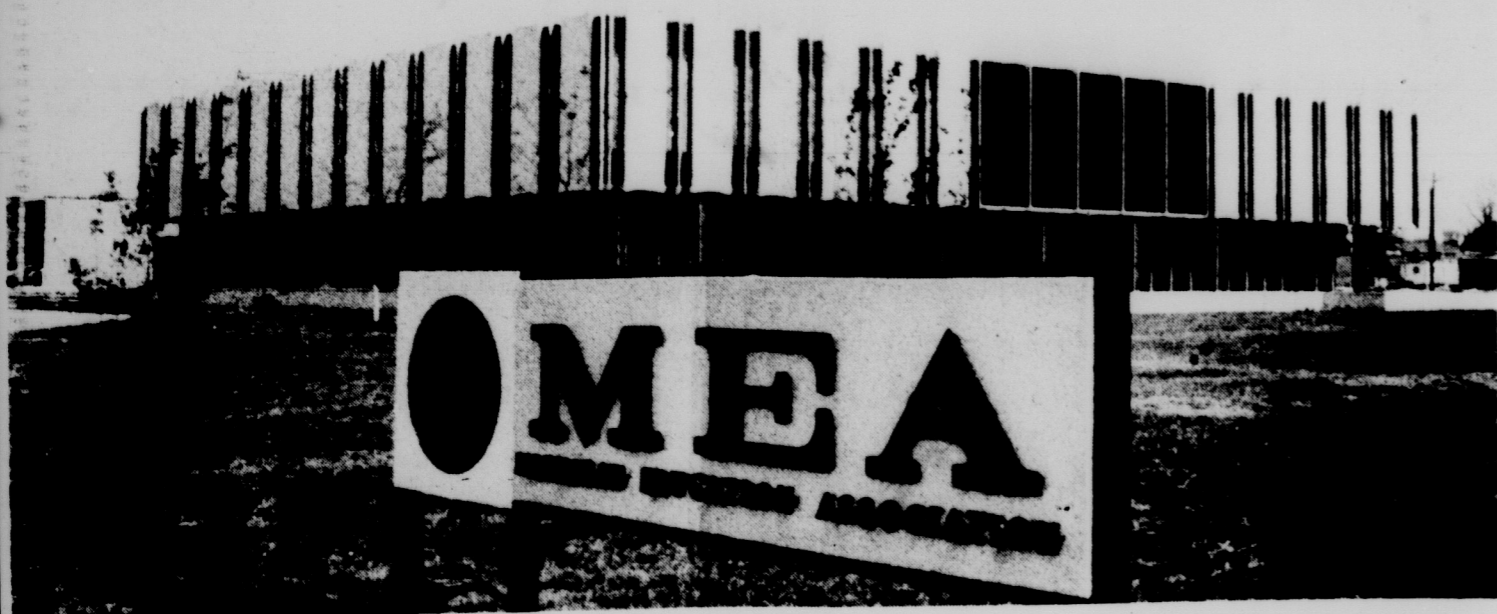
NEW MEA BUILDING DEDICATED--MSU President John A. Hannah recently dedicated the Michigan Education Association's new headquarters located at Abbott Rd. and M-78 in East Lansing.
