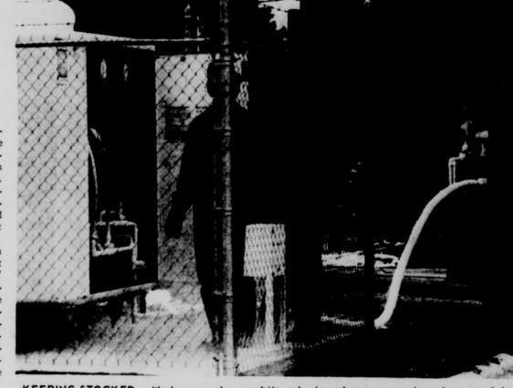
KEEPING STOCKED -- Workers are shown refilling the liquid nitrogen tank at the rear of the Physics-Math Building. The filling line is coated with frost, and the vent tube is giving off a cloud of vapor. Photo by Pete Westerman
