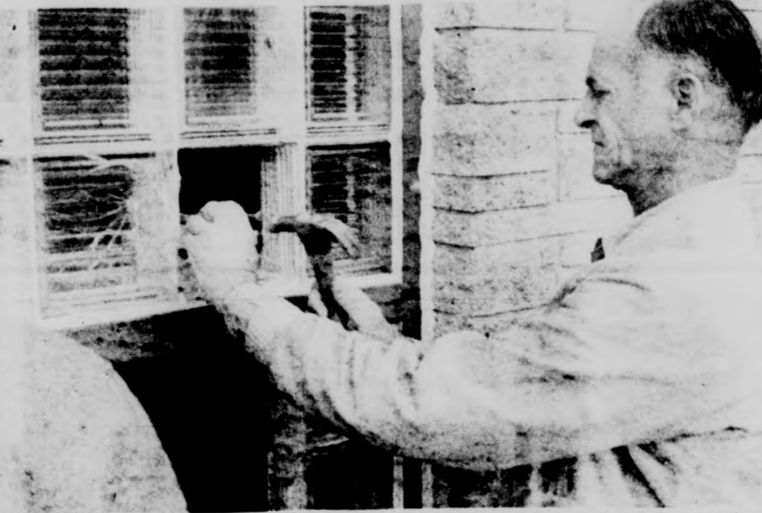
REPLACE BROKEN GLASS BLOCKS—Workmen started the job last week and they say they will be at it until the weather becomes too cold for the mortar to set. There are hundreds of the broken glass blocks still to be replaced in Spartan Village.
