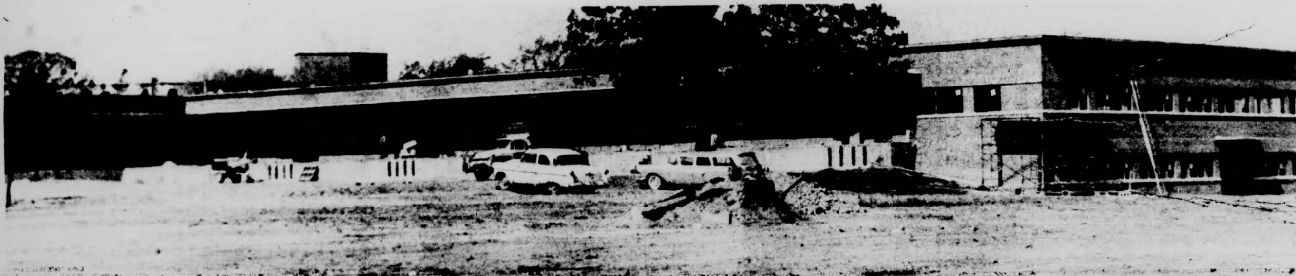
The Physical Plant Department Will Be Centralized In This New $785,000 Structure Scheduled For Completion In Early November
