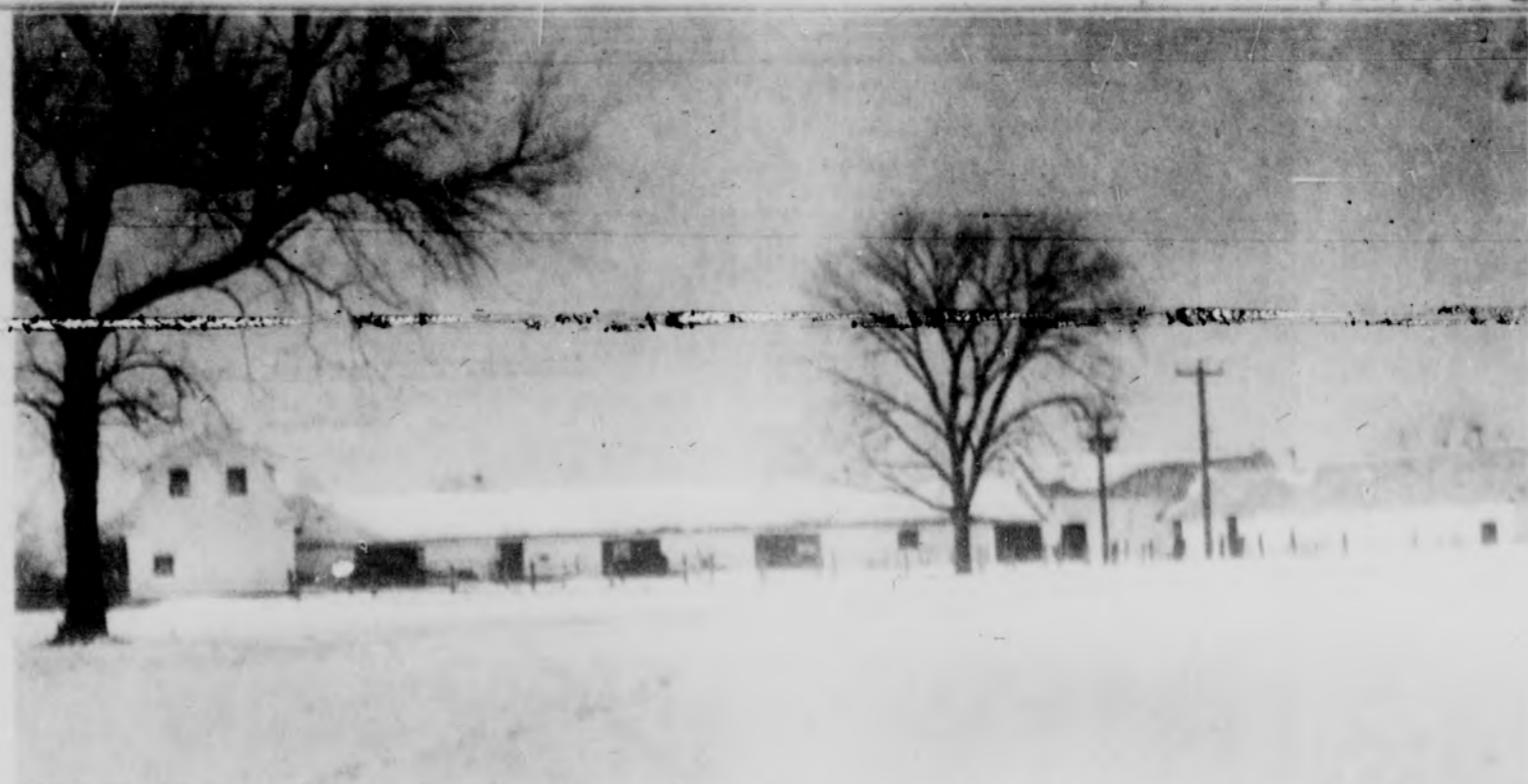
SOON TO GO—South campus will no longer enjoy barnyard smells and shade when this barn, last of the class-building barns, is torn down. Bids for removing the barn, located immediately south of the Engineering building, were received Feb. 5.
