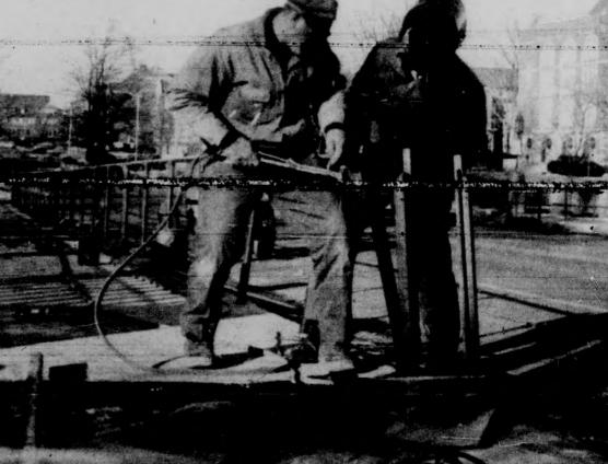
BRIDGE RAILS -- Workmen finish the new rail fence along the Red Cedar Bridge on Farm Lane. The fence will prevent students from inadvertantly stepping into traffic from the crowded sidewalk.
