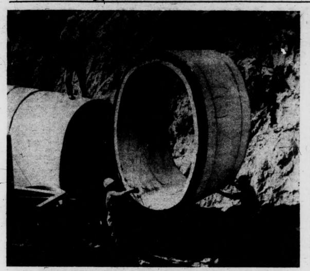
STRONG MEN-Two workers laying the large oval-shaped cement pipe only appear to be lifting the section. In a 25-foot hole along Shaw Lane near Harrison, numerous workers and heavy equipment labor to complete one of the construction projects now taking place on campus.
