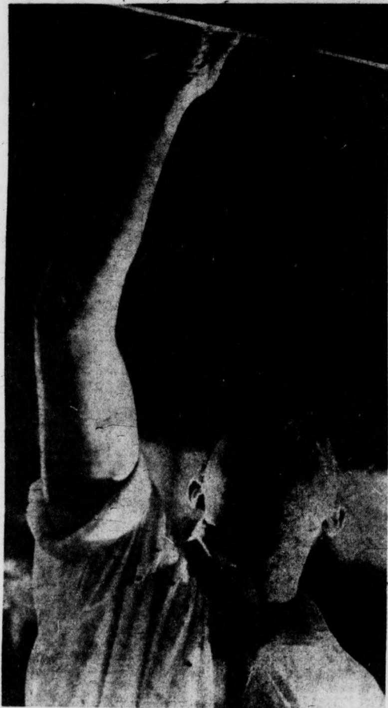
A DOOR in Bessey Hall gets its first coat of paint. The building is to open in the fall.
