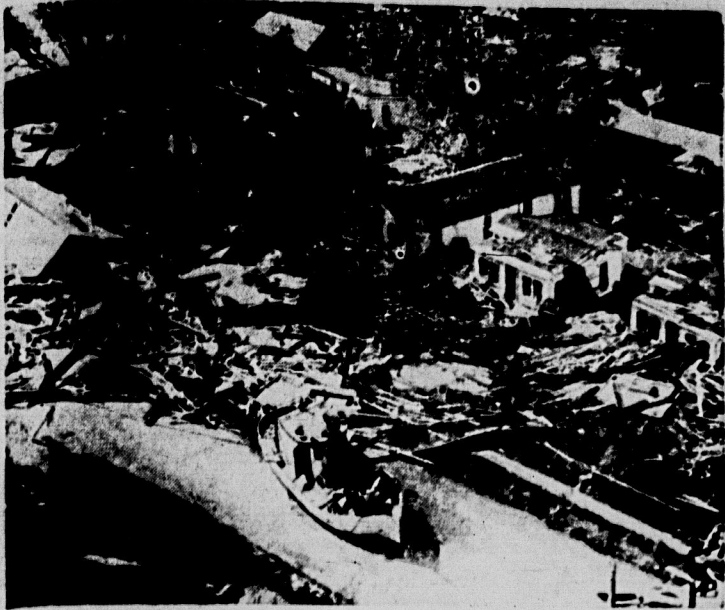
A boat left high and dry on highway next to shattered homes is mute evidence of the fury with which Audrey, first hurricane of 1957, struck the small Louisiana coastal town of Cameron in June. Storm's death toll was more than 500.
