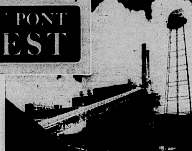
This powerhouse for a nylon plant at Marlinton, Va., was designed by Du Pont engineers. It houses two 135,000 lb. hr. boilers and two 7,000 KW extraction turbine generators.
