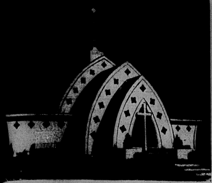
STYLED CHURCH —The new Church Good Shepherd near Kansas City, Mo., reshaped windows, resembles a cross in air. A prefabricated building seating 200 people, it was erected by its Episcopal congregation in the equivalent of seven working days.
