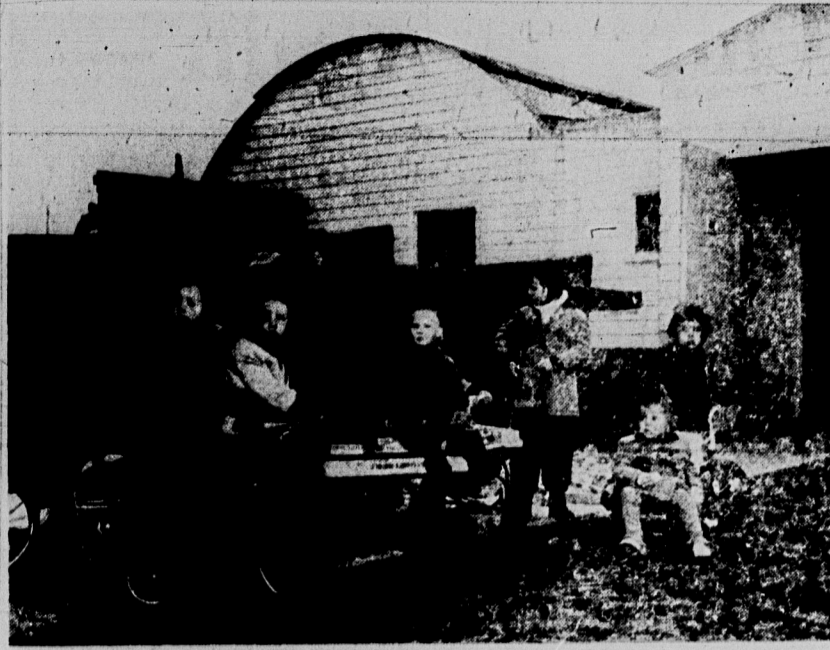
Nursery Director Elizabeth Page supervises some of her future charges as they watch construction of the MSC nursery to be completed.
