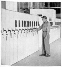
**POWER**—Neat, compact and safe switchgear installation is big improvement over open framework and knife switches in older installations,
