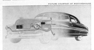
In its regular pattern of functioning, an oncoming car moving with its "brights" engaged, would cause the device to undergo a switching-action as soon as it appears on the device's horizon." Your headlights automatically go from bright to dim—stay that way until all oncoming traffic passes. When the opposite lane is clear they automatically return to bright.
