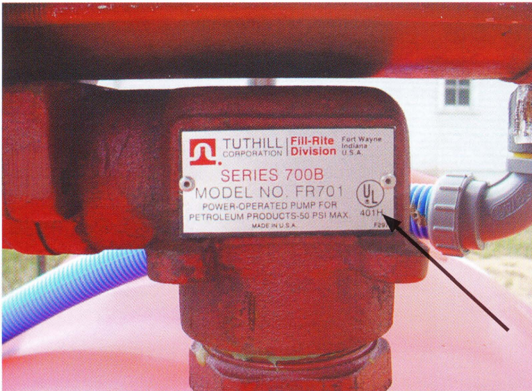
Fig. 9. Tanks and equipment must meet Underwriters Laboratory (UL) standards for the type of fuel and usage. Check the label.
