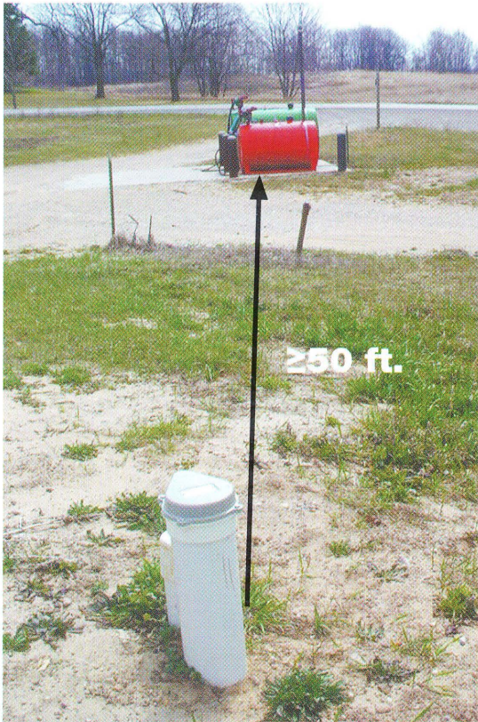
Fig. 3. Fifty-foot separation distance between private drinking water well and fuel tanks. Greater distance needed for Type III or Type IIb public well (dairy farm or farm with employees).
