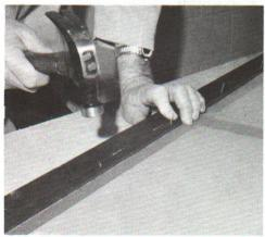
Step 7. Nail or staple the screen fabric on all four sides of each panel about every 4" to 6". Work from center to each end to prevent a bulge from developing.
