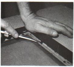
Step 2. Remove the old screen material by taking out the tacks or staples.
