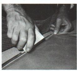
Step 3. Spread the screening over the frame and press the retainer strip into the groove.
