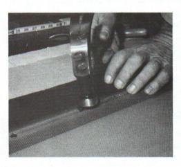
Step 4. Attach the new screen fabric at one end with regular ½" carpet tacks. A stapler works well, also.
