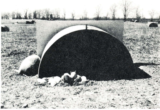
Quonset shelter for field farrowing.
