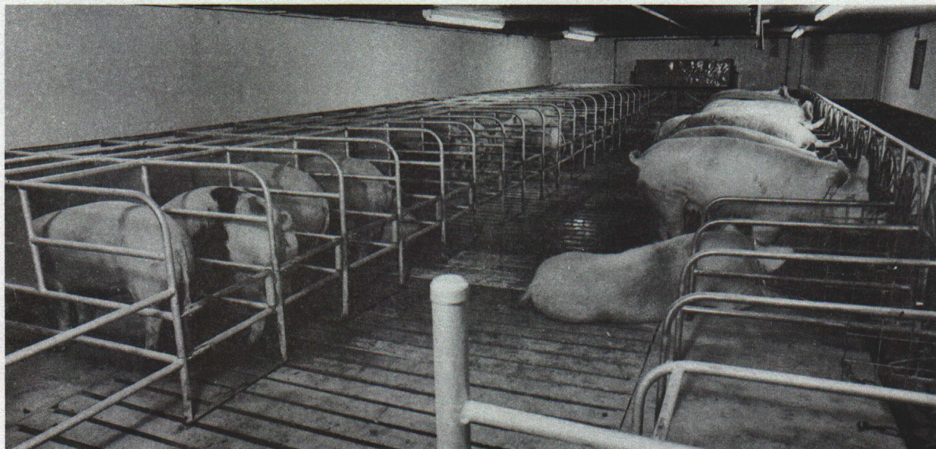
IN THE FLUSHING SYSTEM at the MSU Sow Gestation barn, the two rows of sows stand with their hind legs on an 8' slotted floor. The front part of the stall is a solid strip of concrete.
