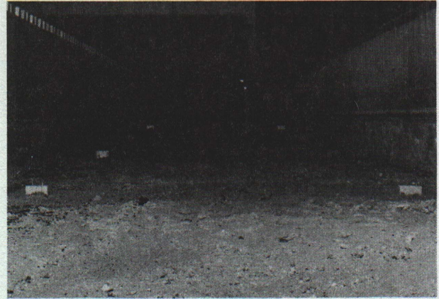
Fig. 5. Stakes in place to give a 2% slope to the floor of the trench.
