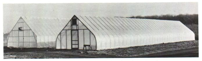
Flexible plastic film can be used for many types of greenhouse construction.
