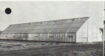
Fig. 4 Completed rigid frame greenhouse.
