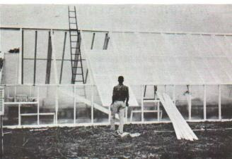
Fig. 5 Installation of the panels that rest on the sash supports.
