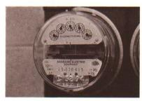
Electrical systems have a *meter* to measure the *amount* of electricity used. The meter records how much work the electricity did for you during the month, and you are billed accordingly. This work is measured in *kilowatt-hours*. One kilowatt-hour of electrical work will probably cost between  $1\frac{1}{2}$  to  $2\frac{1}{2}$  cents and will light a 100-watt bulb for 10 hours.
