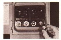
Adapters come in different sizes according to the amperage of the fusestat. A 15-amp adapter will accept only a 15-amp fusestat. Once the right adapter is screwed into the fuse box, it cannot be removed and only fusestats fitting that adapter can be inserted in the fuse box. This simple safety measure prevents needless fires due to using the wrong fuse size. It is especially useful in preventing overloads in cottages or other rental properties.
