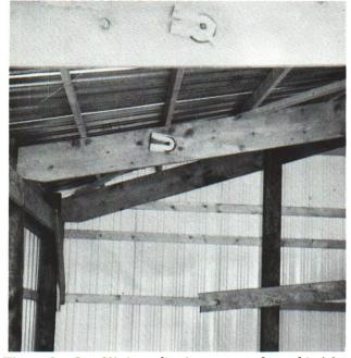
Figure 2 – One-2<sup>1/2</sup> in. split ring was used on this joint where at least two rings should have been used.
