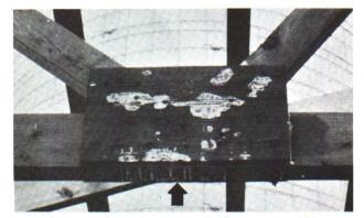
Figure 5 – Evidence of a well-filled glue joint – glue running down the side of the  $2 \times 4$ .
