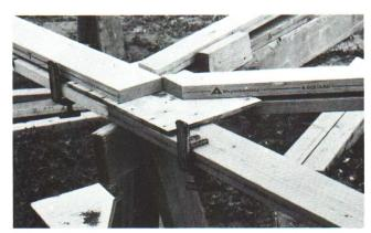
Figure 3 – Use one truss as a pattern. Cleats nailed to side of pattern truss facilitate assembly.
