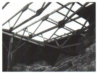
Figure 11 – Poor nailing of roof girts to trusses caused this section of roof to blow off during high wind.
