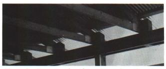
Figure 8 – Truss to rafter-plate joint made with a short 6 in. by 6 in. block.
