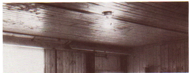
Figure 7 — A continuous slot inlet along the edge of the ceiling allows fresh air to enter (above). A hinged door helps direct the cold air along the ceiling and become warmed before dropping on the small calves. A fresh air inlet in the ceiling over an alley (below).
