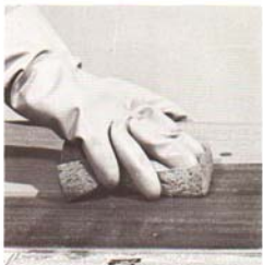
Apply bleach solution with a sponge. Be sure to cover the area completely.
