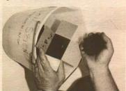
Place a pint of the soil in a clean container for transferring to the soil testing laboratory.
