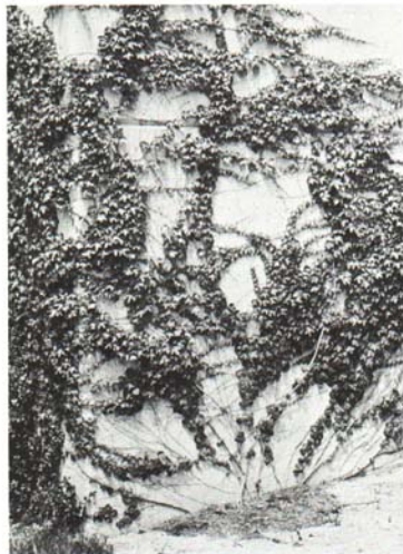
Fig. 13. Veitch Japanese Creeper climbing on masonry building.
