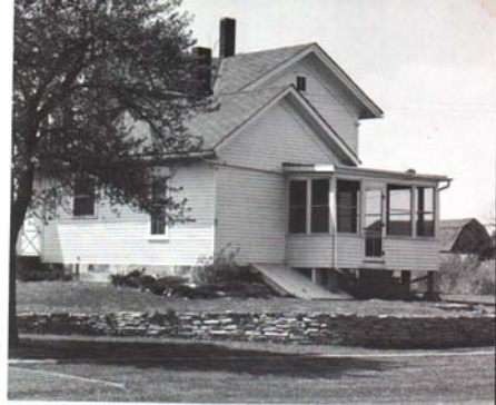
Fig. 32. Walls offset disturbing height and may be constructed without mortar if allowed to slope toward higher ground. Plants could be used to reduce the bareness of this back porch.
