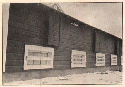
Fig. 9.—Rear Elevation—note the rear windows and the construction of the intake flues.
