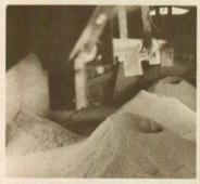
Conage is transferred daily from silo storage to floor above milking patric and cropped in piles over large down chutes to milking stalls. Some gravity flow takes place as shown by holes in center of each grain pile. Operator must rebuild piles over down chutes after each milking. Closed automatic feeding systems that depend on pressure switches for operation do not work satisfactorily as the high moisture material tends to build up and bridge when under pressure.
