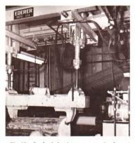
Fig. 16. Overhead charging crane to service the cant gangsaw. Here it is being used as a lathe charger and is considerably heavier than required for stacking cants on the gangsaw infeed table, but it illustrates the principle. The design of the crane permits precise alignment of the cant for maximum lumber yield. By stacking the cants in multiples of four, the gangsaw can easily keep up with the production of the pole mill. (Photo: Edeher Engineering Co.)
